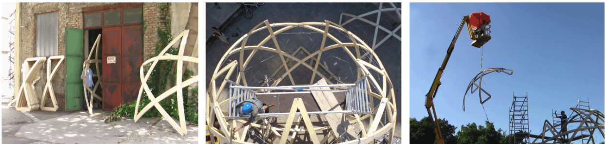
Figure 11: Construction scenes: left, component prefabrication in university workshop; center/right, on-site assembly in Viennese park adjacent to university and church of St. Carl.
